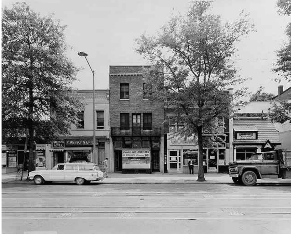
100 block Independence Avenue SE (May, 1962; U.S. Architect of Capitol, via Library of Congress)
